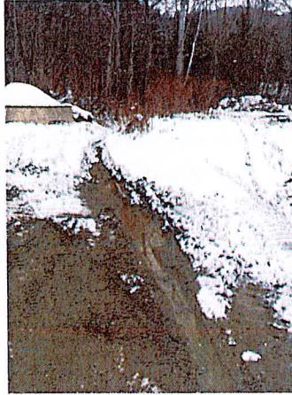
Drainage from the sand storage facility by the entrance is entering a swale that drains to the Mad River.
